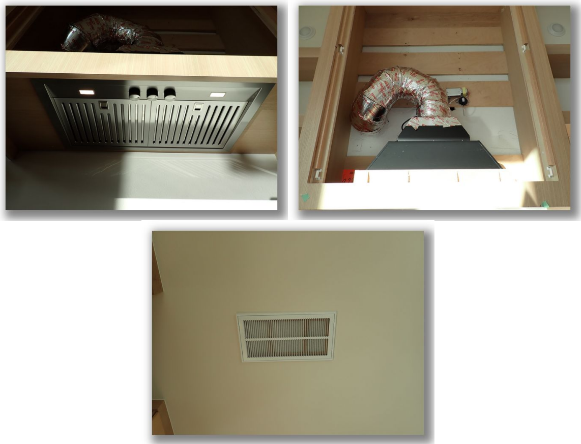
Butler's Pantry Range Exhaust Systems All components were found to be performing and in satisfactory condition on the day of the inspection.
